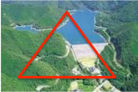
Hydroelectric power plant
