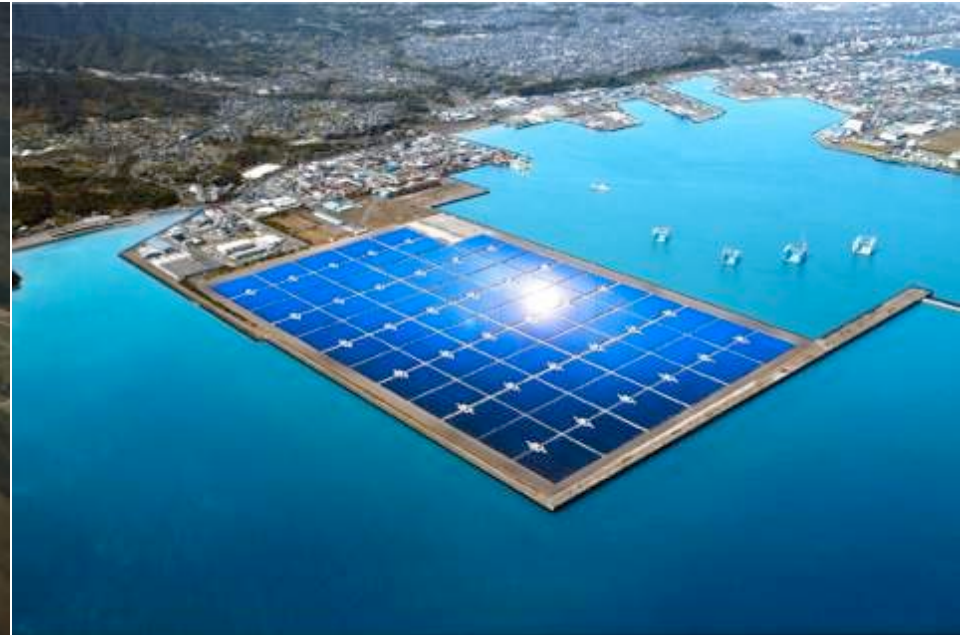
70 MW Power Plant in Kagoshima, Japan
