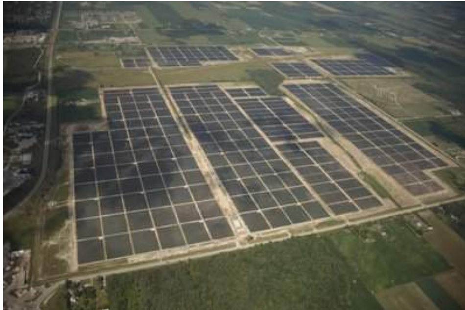
80MW Power Plant in Canada (World largest, 2010, 1km 2 approx.)
