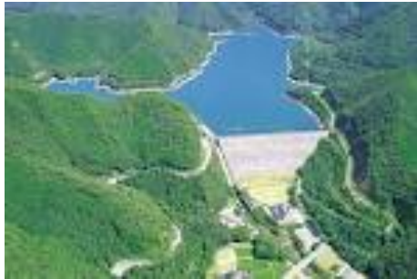
Hydroelectric power plant
