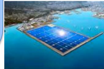
Solar power plant on ground
